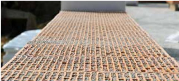
The granules are filled into the cavities of the brick!
