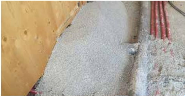
2nd step GEOMATERIALS expanded glass covers all installation lines
