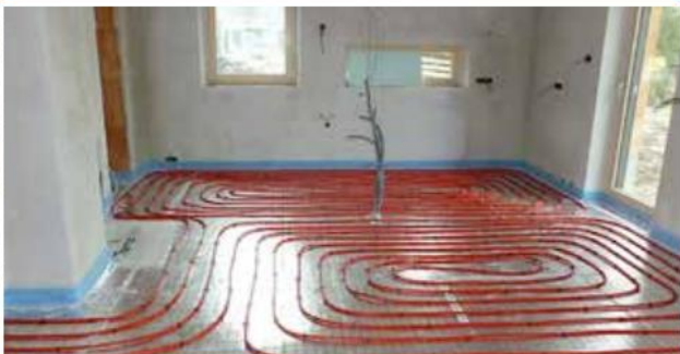
Step 6 - Laying underfloor heating After the drying time of at least 48 hours
