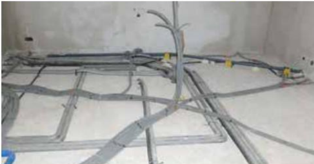
1st step - rough installation Completed installation work before thermal insulation
