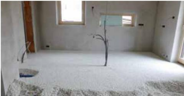
Step 3 - Install insulation fill level and level down to the intended level
