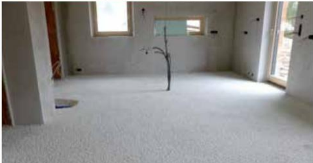
4th step - fully installed all installation lines are seamlessly encased and thus isolated
