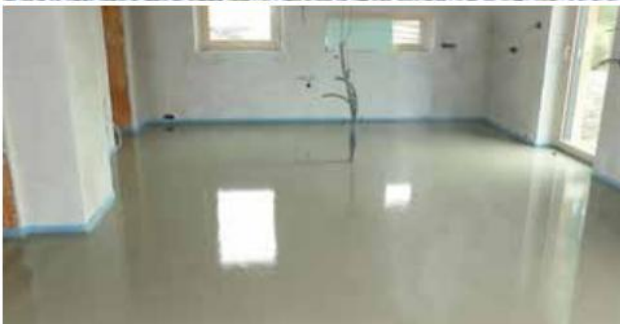
Step 7 - Screed is installed at the desired level according to the plan
