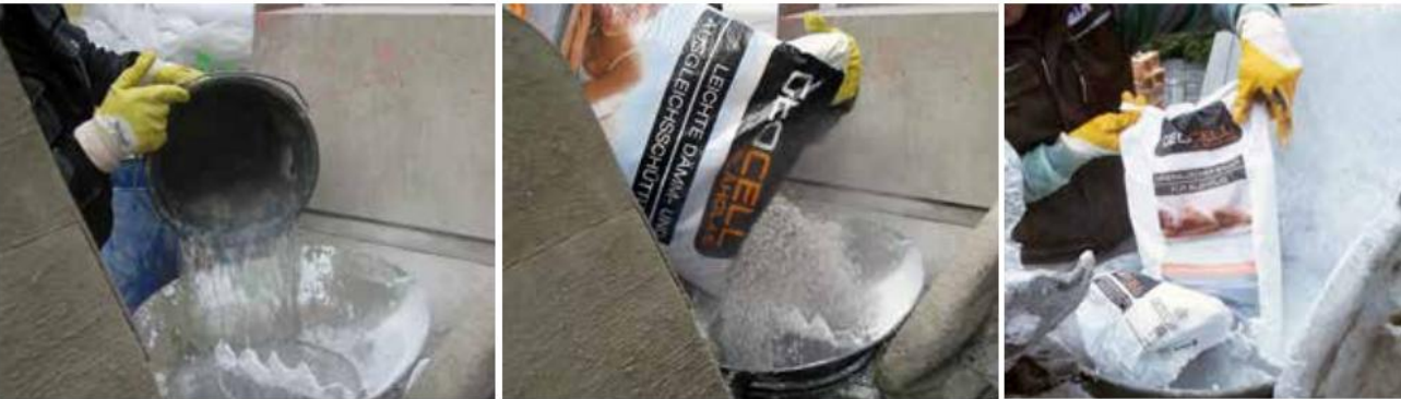
Water as needed (may vary depending on mixer performance vary) GEOMATERIALS expanded glass GEOMATERIALS mineral Binder
